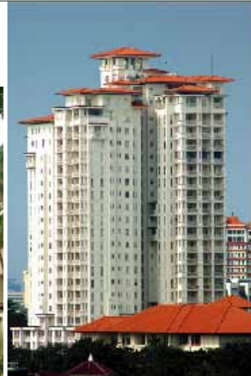
Dharmawangsa Hotel & Apartment, Jakarta
